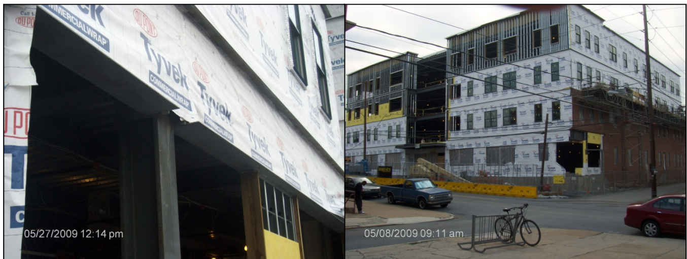
Figure 1 – Masonry Façade Steel Support Angles
